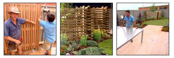
**Barbecue bench:** A Murrary River Redgum bench top (which was made from a salvaged fallen tree) was placed on top of a 90x45mm treated pine frame which was then faced with treated pine battens and oiled. A bench top barbecue was measured and an appropriate opening was cut in the bench top for fitting.
